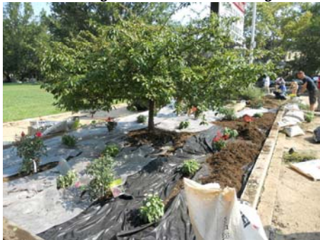
Laying the weed guard and flowers
